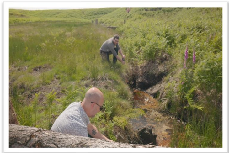
Prof. Mark Trigg and Dr Tom Willis measuring a leaky dam as part of the Backstone Beck project.
