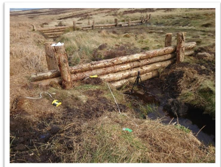
Leaky dam NFM on Backstone Beck on top of Ilkley Moor
