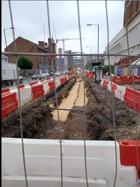
Housing Zone North - 20 SuDS cells under construction
