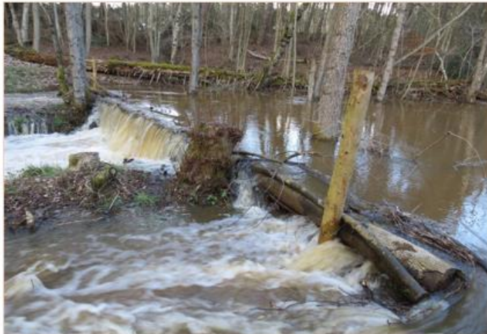
(Leaky Dams installed on Pickering Beck. Photo: Nick Odoni)
