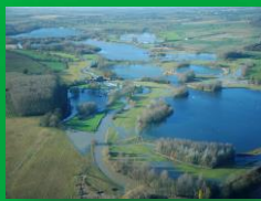
In-channel measures to restore river floodplain connection
