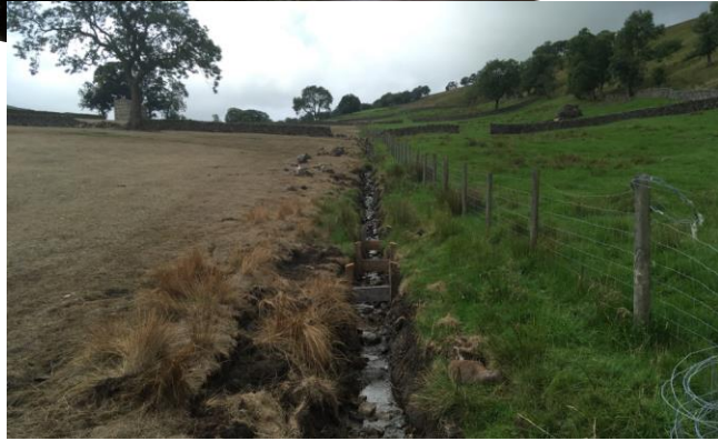
De-culverting
